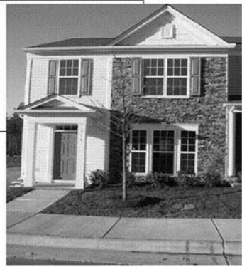
It's important to keep up with the maintenance ... an ounce of prevention or attention now saves angst & dollars in the future
